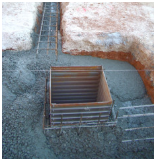
1. Placement of the CUBIX into the reinforcement.
