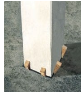
3. Place the column in the foundation and fill in the clearance of the filling material.
