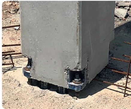
Column placement and screwed.
