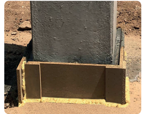
Joint filled with GROUT mortar.
