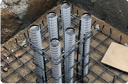
Sleeve placing.
