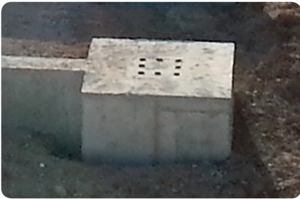
Prepared support for placing the column.
