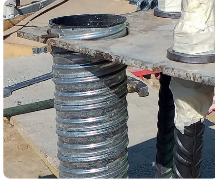
Sleeve with cap - bolt - template detail.
