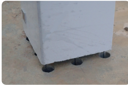
Reinforcement placed inside the sleeves.
