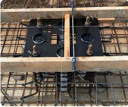
Sleeves and TN anchor bolts placement.
