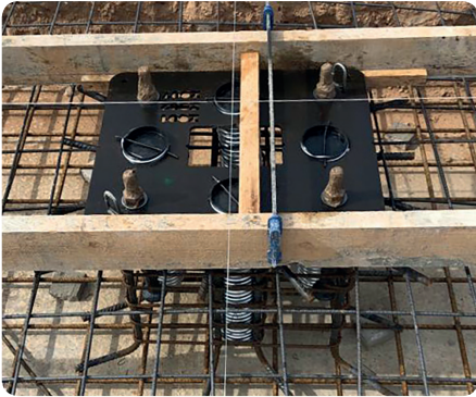
Sleeves and TN anchor bolts placement.
