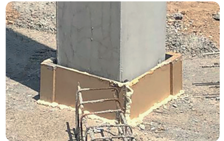
Preparation for filling the joint with GROUT mortar.
