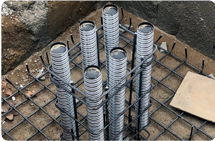
Sleeve placing.
