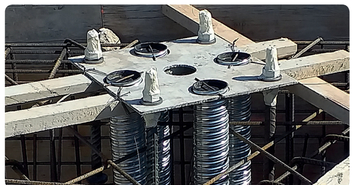
Prepared template for the concrete pouring in the construction site.
