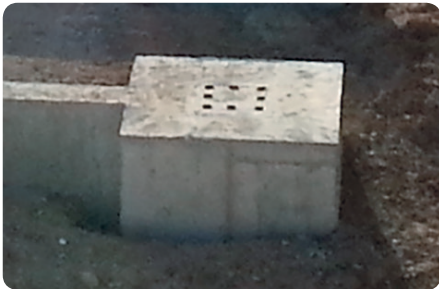
Prepared support for placing the column.
