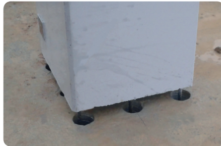
Reinforcement placed inside the sleeves.
