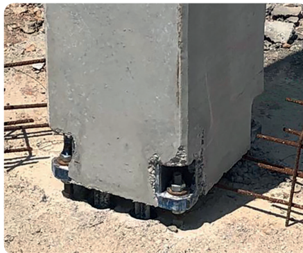
Column placement and screwed.
