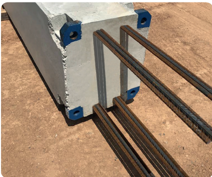
Column prepared for the assembly.
