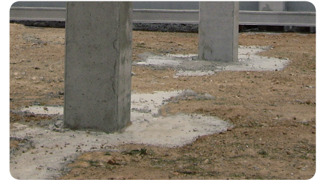
Joint concrete pouring.
