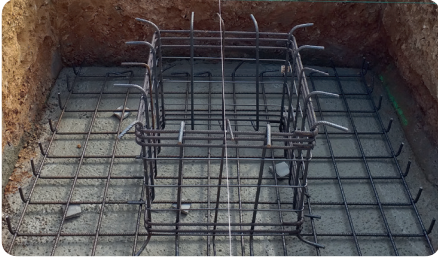
Excavation and reinforcement preparation.
