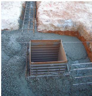
1. Placement of the CUBIX into the reinforcement.
