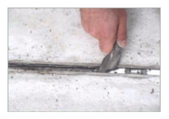
2.1.- Remove the polystyrene protection, if desired. (Accessories can be inserted without removing polystyrene)
