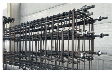
Long bolts inserted in a column reinforcement.
